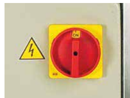
FVG - Main switch for emergency stop FVG - Notschalter
